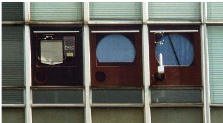
Figure 2: The four driving rain gauges on the west facade. From left to right: TUD, CTH, TUE-I and TUE-II. An ultrasonic anemometer has been mounted below TUE-II.
