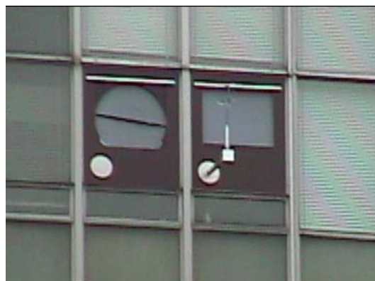
Figure 2.6: Driving-rain gauges in the west facade of the Main Building at position P5 (left) and P4 (right).
